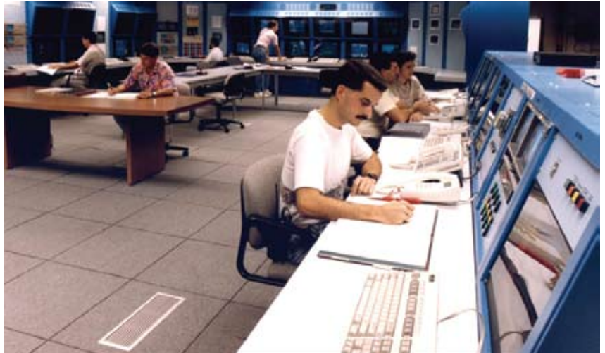
Machine Control Center (MCC)
